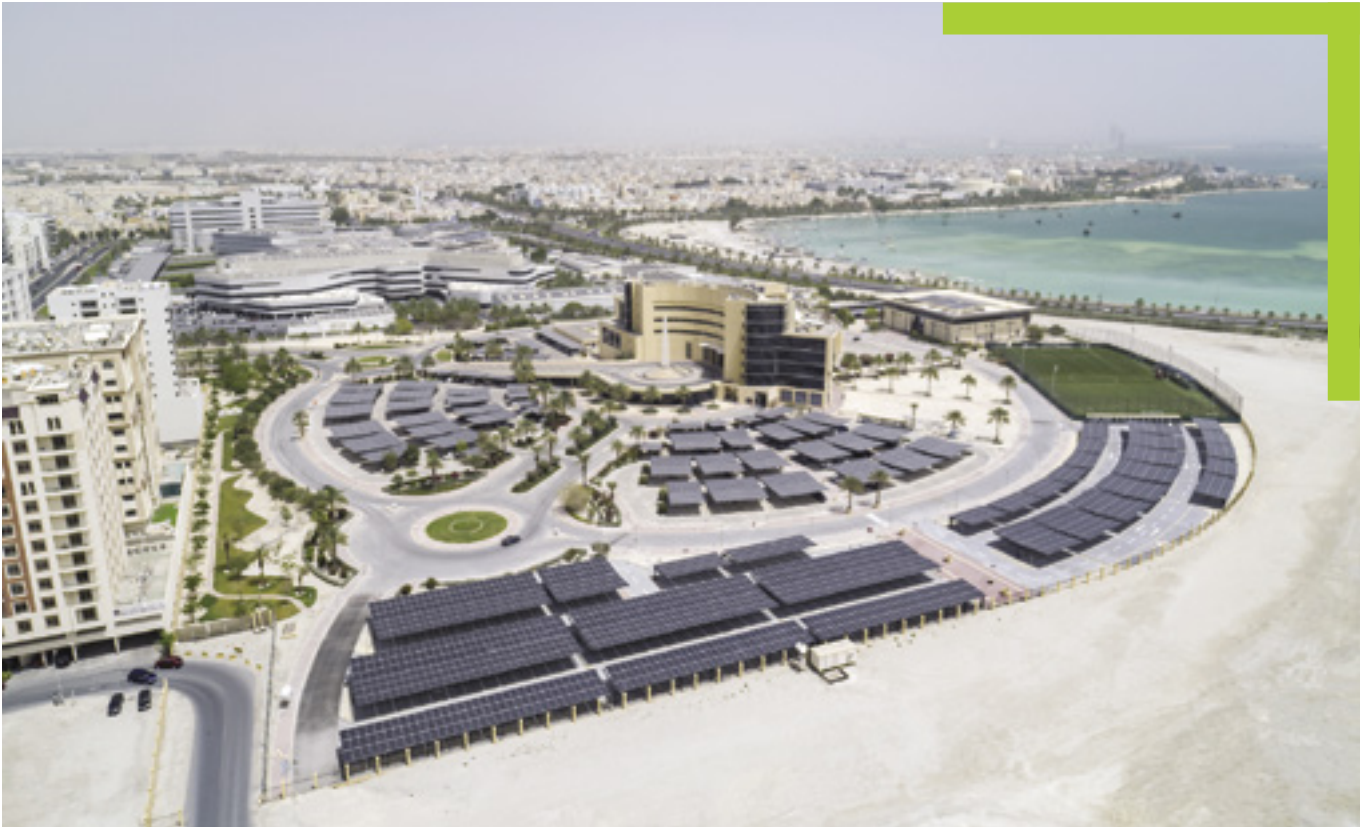
RCSI Bahrain's Solar Project will cover approximately 65% of the university's annual electricity needs
