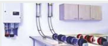
BEST HOSPITAL SUPPORT SYSTEM Automatic Medicine & Sample Delivery System from Pharmacy to ICUs, Wards, OTs through Pneumatic Tube
