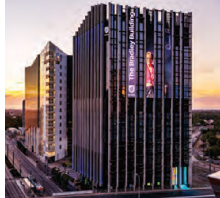
Located in Adelaide's BioMed City, the Bradley Building is a leading destination for health research and teaching. It's home to one of the most significant concentrations of cancer researchers in the state, and features the latest tools and technologies to support improvements in patient diagnostics and treatments.
